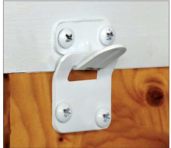
Fig. 1 Here the Norse hook and hanger supports a plywood panel mounted flush inside the window frame.
