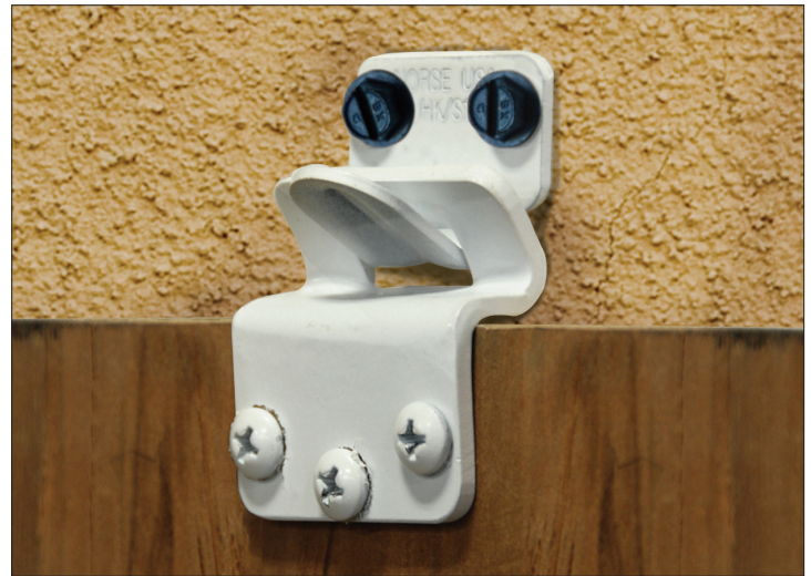
Fig. 1 The Norse hook and hanger supports a plywood panel surface-mounted against the window frame face
